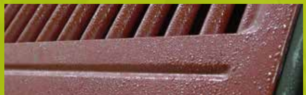
Condensation on components due to changing conditions
